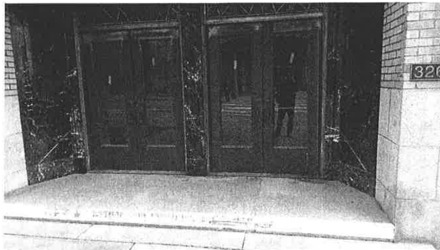
Figure 3: Main Entry Doors
