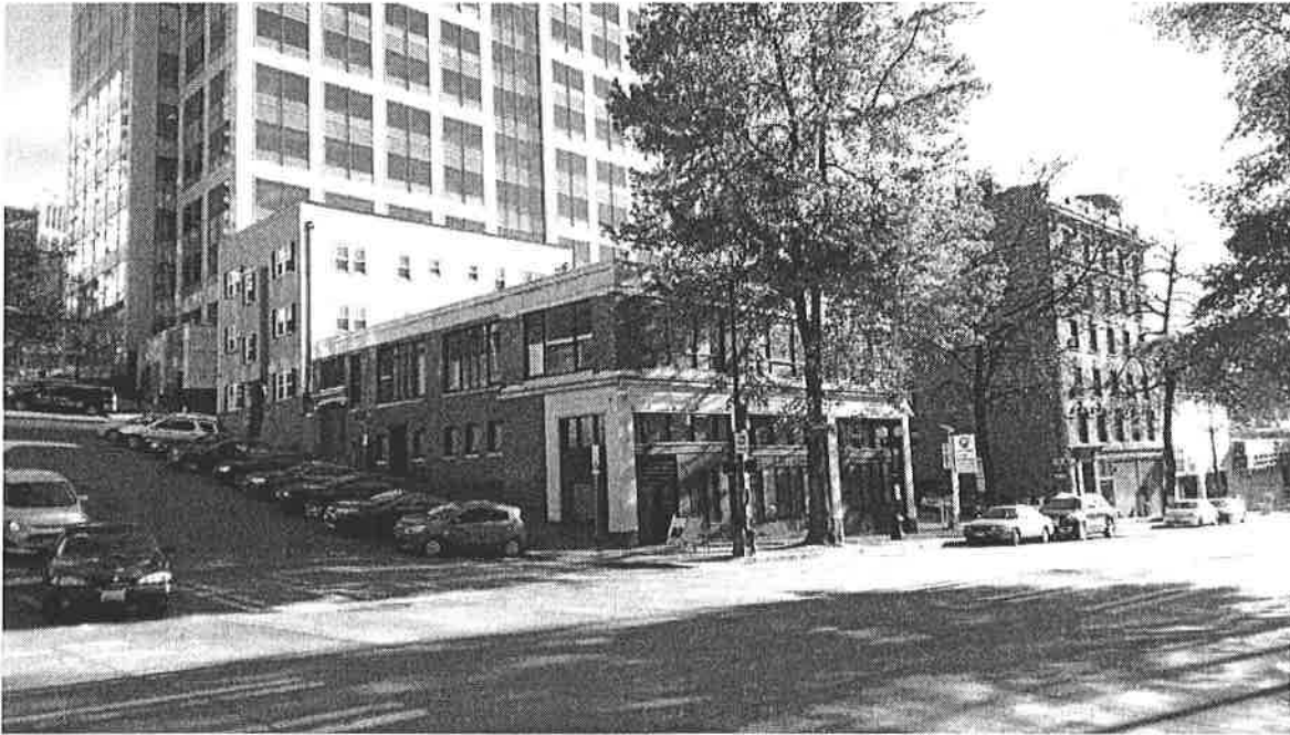
Figure 4 -Exterior: view from north-west corner of 4th Ave. & Jefferson St.
