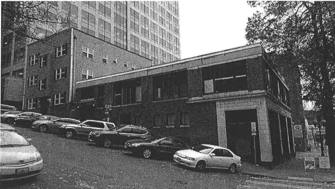
Figure 5 – Exterior: Facade along Jefferson St.
